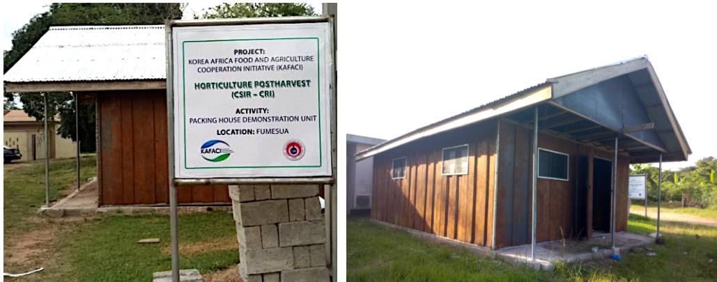
Figure 3. Demonstration Pack house unit under construction at Fumesua Station
